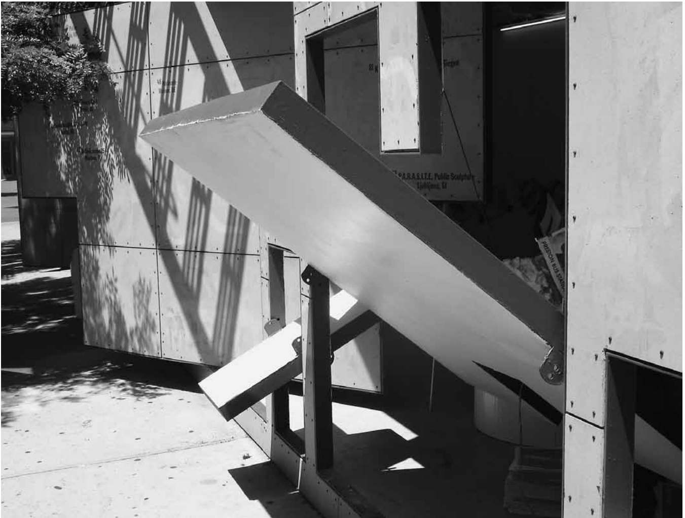
Figure 3. Acconci Studio. The Storefront for Art and Architecture , New York, 1993. Post-2008 reconstruction (Photo: A. Forster).
